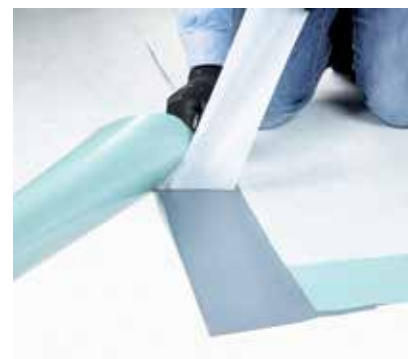
Sealing by butyl tape RENOLIT ALKORPRO BAND .
