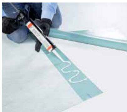
Sealing by mastic glue RENOLIT CEM 805 .
