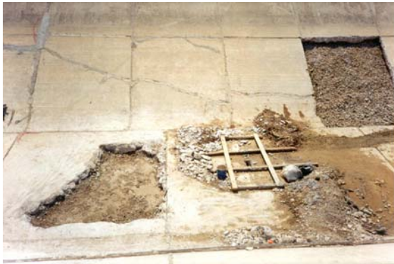
Repair of old canal bed and cleaning of sub-grade
