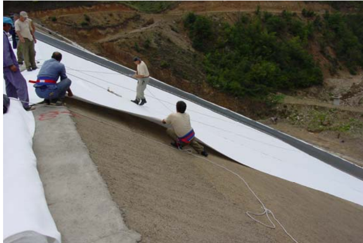
Placing of geotextile
