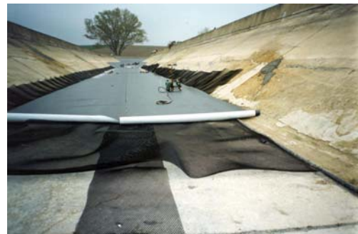
Unrolling and placing of geomembrane
