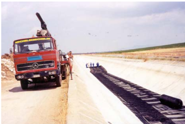
Geo-grid as drainage under waterproofing
