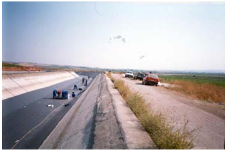
Welding with hot air and double seam
