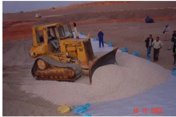
Distribution of material with bulldozer
