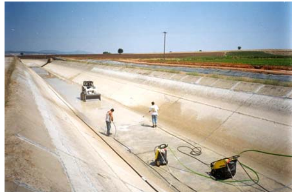
Repair of old canal bed and cleaning of sub-grade
