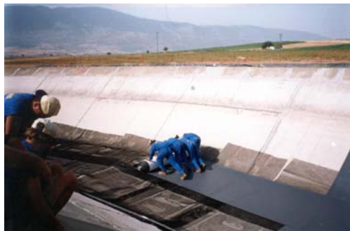
Unrolling and placing of geomembrane
