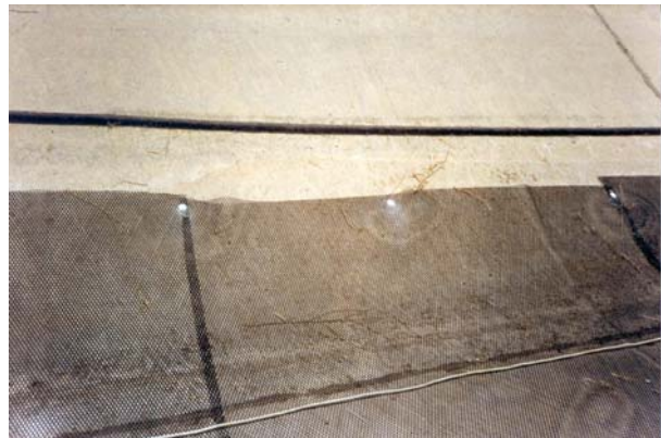
Geo-grid as drainage under waterproofing
