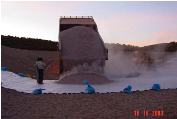
Unloading of protection material with truck
