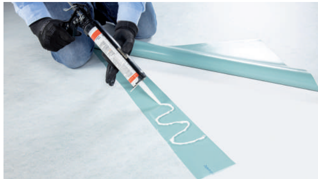
Sealing by mastic glue RENOLIT CEM 805
