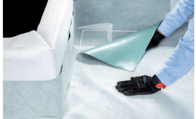
The corners and angle areas are sealed using pieces of membrane RENOLIT ALKORPRO shaped and sealed with the RENOLIT CEM 805 mastic glue.
