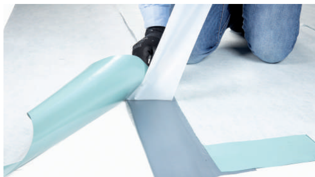
Sealing by butyl tape RENOLIT ALKORPRO BAND
