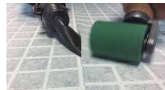
Overlap welded seams
