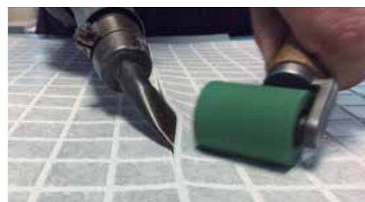
Butt welded seams
